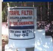
Community Terafil water filter(1000 lit. day capacity)
